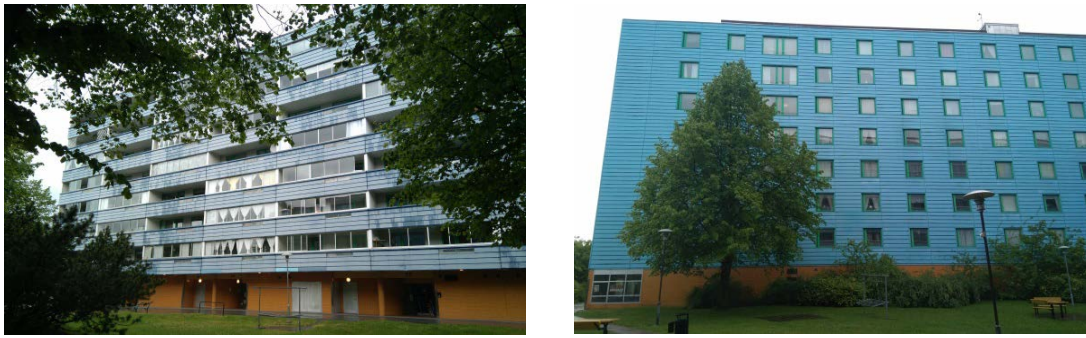
Figure 2.2-4: Front façade (left) and back façade (right)
