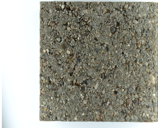
Figure 3.1: Picture of an old, already carbonated, Portland concrete specimen
