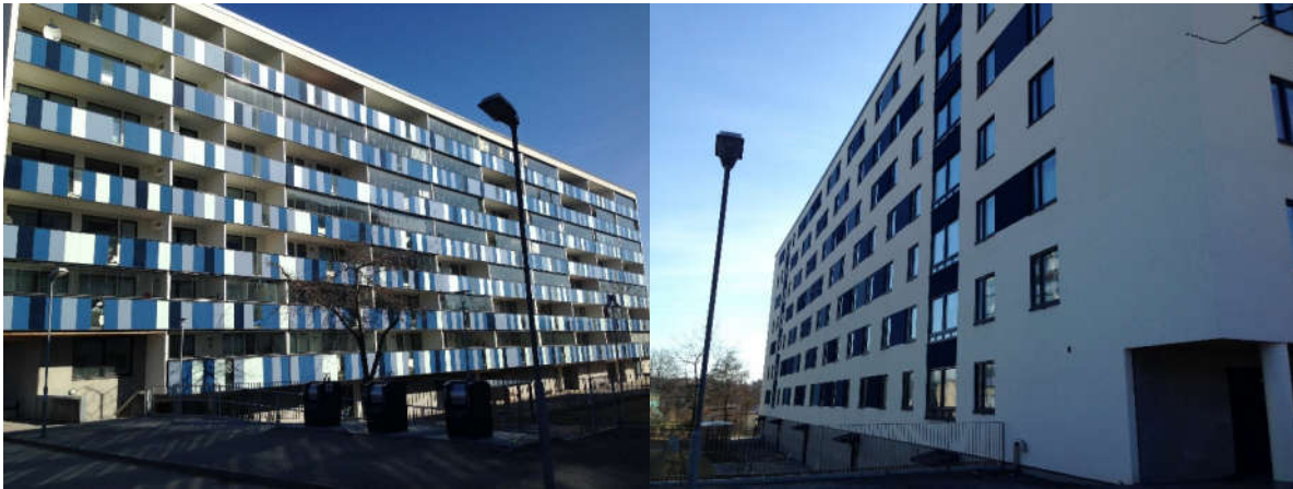
Figure 3.1.3 Facades of renovated building. south (L) and north (R).
