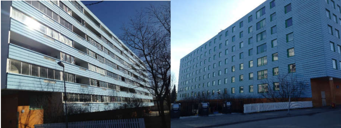
Figure 3.1.1 Facades of nonrenovated building. south (L) and north (R).
