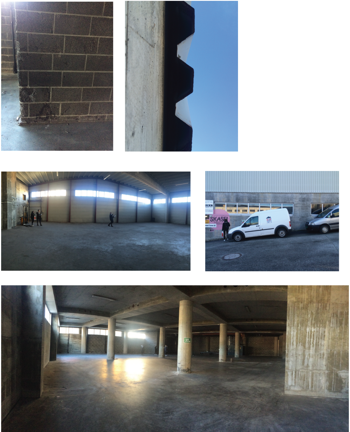
Figure 15: Site pictures of the warehouse
