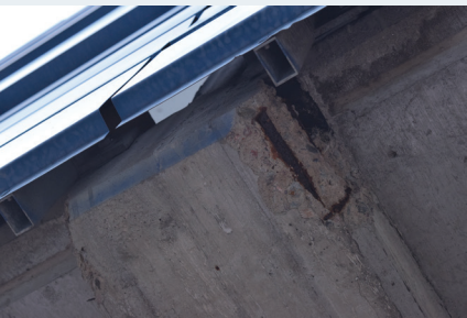
Rebar protruding
